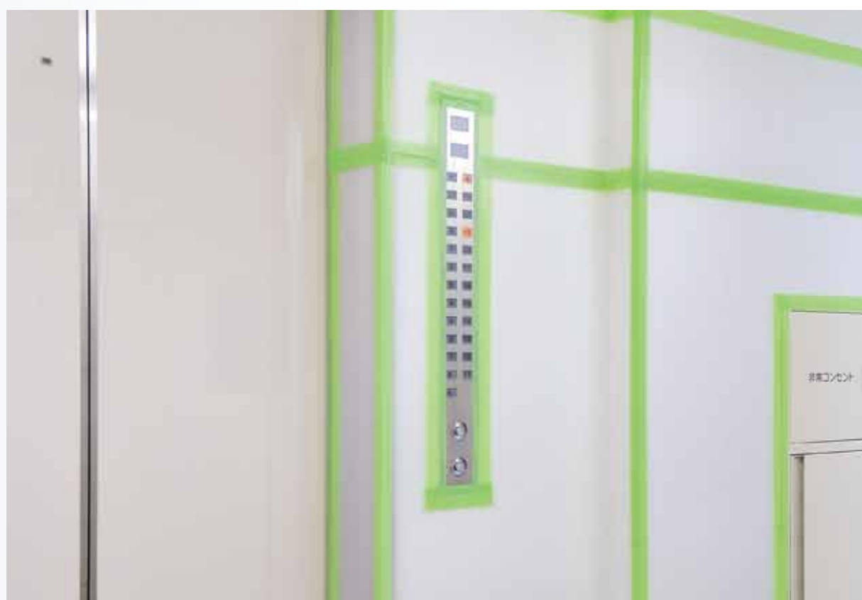
養生用(室内) Indoor masking.
