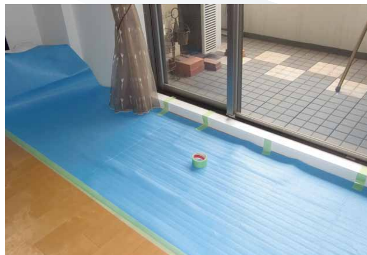
養生用(室内) Indoor masking.
